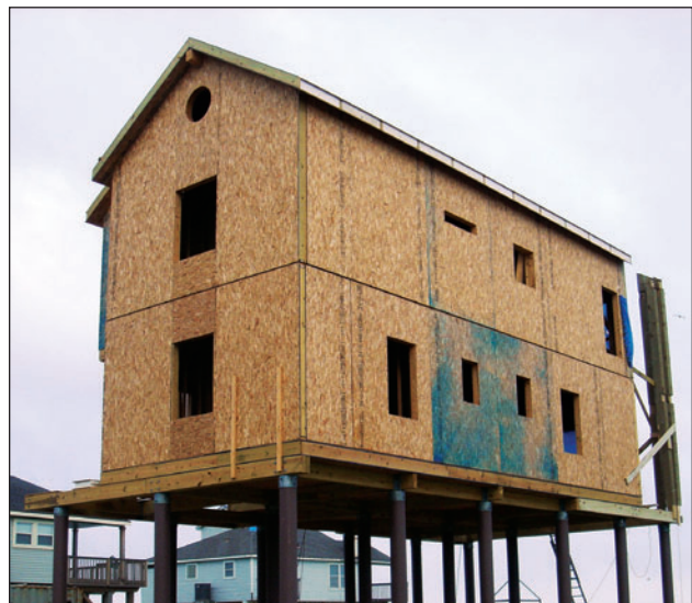
Figure 2. Construction of a Structural Insulated Panel house.
