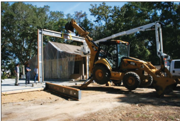
Figure 4. Installation of a prefabricated ordinary moment frame.
