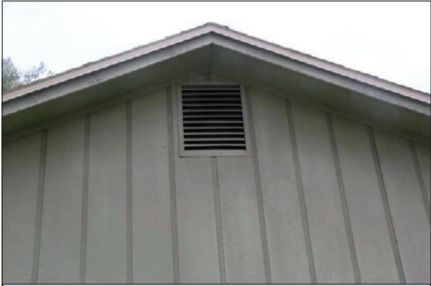
Figure 9. Gable end vent.
