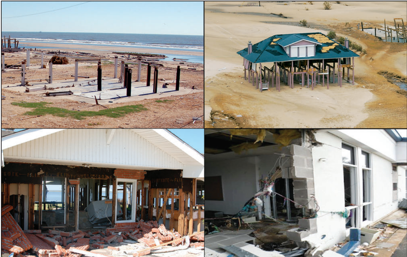
Figure 5. Hurricane Ike damage to buildings. The upper left and upper right photos are of buildings that were close to the Gulf of Mexico shoreline and subjected to storm surge and large waves above the lowest floor. The lower left photo is of a building close to Galveston Bay shoreline and subjected to storm surge and small waves. The lower right photo is of a Cameron Parish, Louisiana, school that was approximately 1.3 miles from the Gulf shoreline, but subjected to storm surge and small waves.
