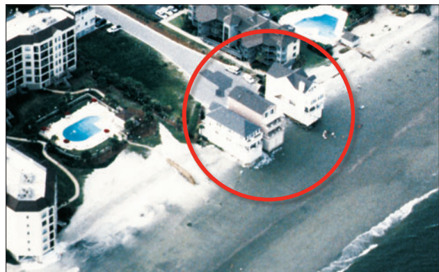
Figure 1. Well-built but poorly sited building.
