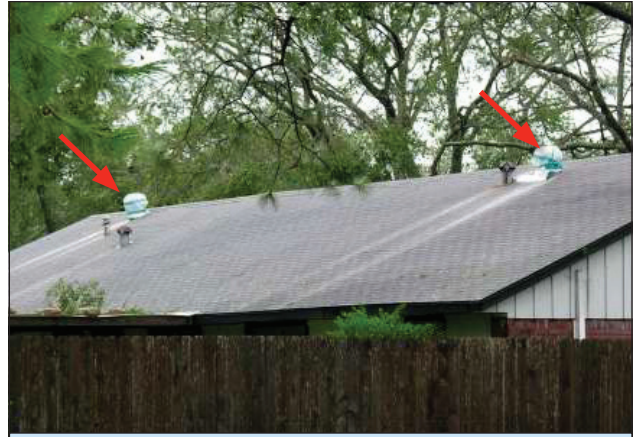
Figure 14. Plastic wrapped turbines.
