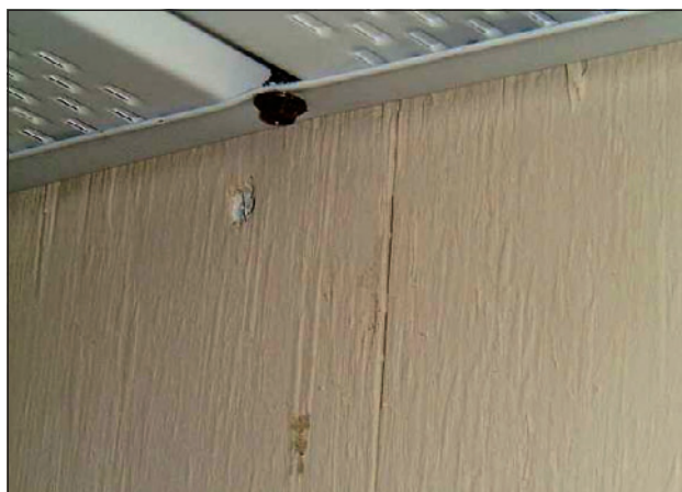
Figure 5. Screws through wall channel.
