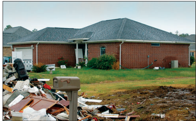
Figure 1. Bridge City, Texas, homes were flooded during Hurricane Ike, even though they were constructed outside the SFHA and in Zone B. The flood level was approximately 4' above the closest BFE.
