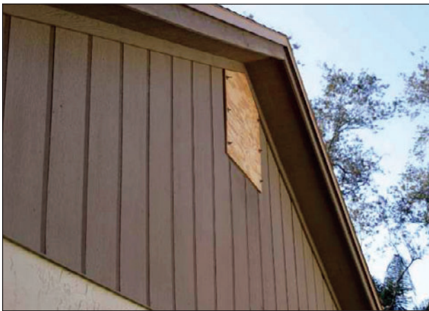
Figure 10. Shuttered gable end vent.
