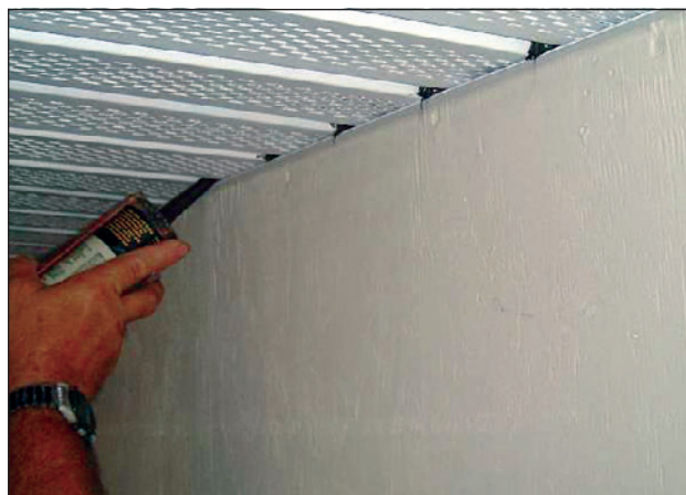
Figure 4. Applying dabs of sealant.
