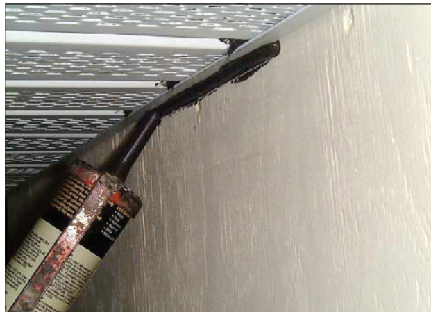
Figure 3. Applying a bead of sealant. (Note: Black sealant was used so that it would be visible in the photograph. Normally a matching sealant color would be used.)
