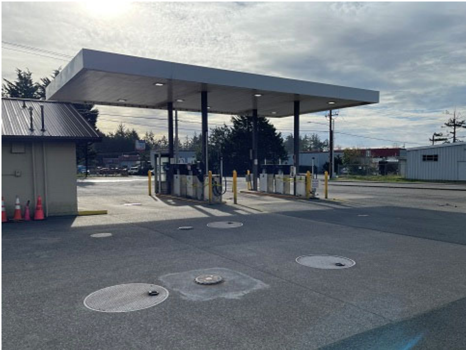
817 NE 3 rd Street – SW View
