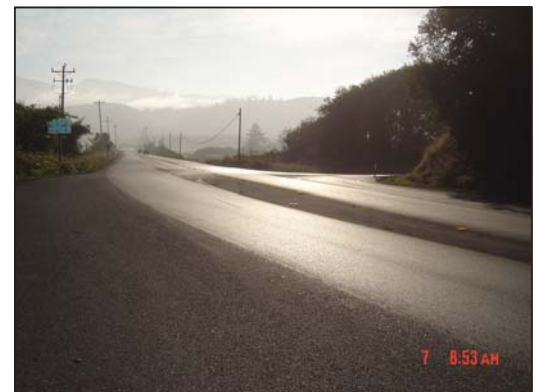
Northbound US 101 Approach
