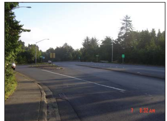
Northbound US 101 Approach
