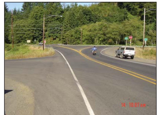
Northbound Business 20 Approach
