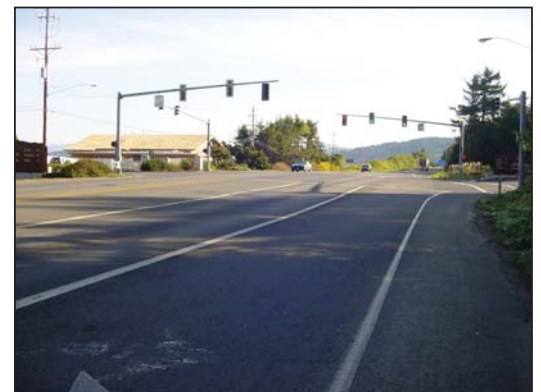
Northbound US 101 Approach
