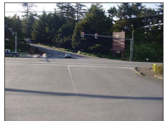
Eastbound Salishan Drive Approach
