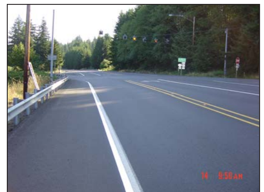
Eastbound US 20 Approach
