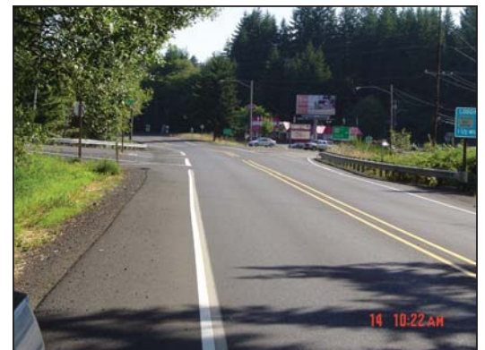
Eastbound US 20 Approach
