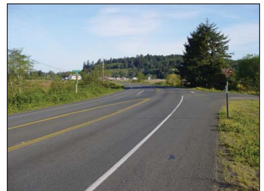
Northbound US 101 Approach
