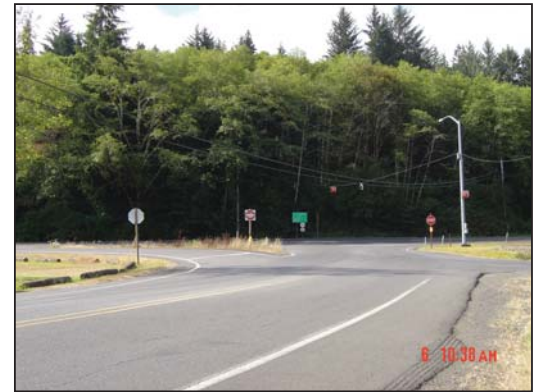
Southbound Old Scenic Highway Approach
