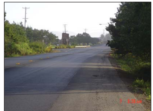
Northbound US 101 Approach
