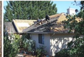
Keep vegetation away from windows and from touching your roof.
