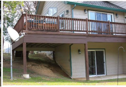
Keep your roof, gutters, and areas under decks clear of needles, leaf litter, or other flammable materials.
