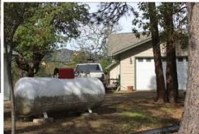
Remove all debris from around propane tanks.
