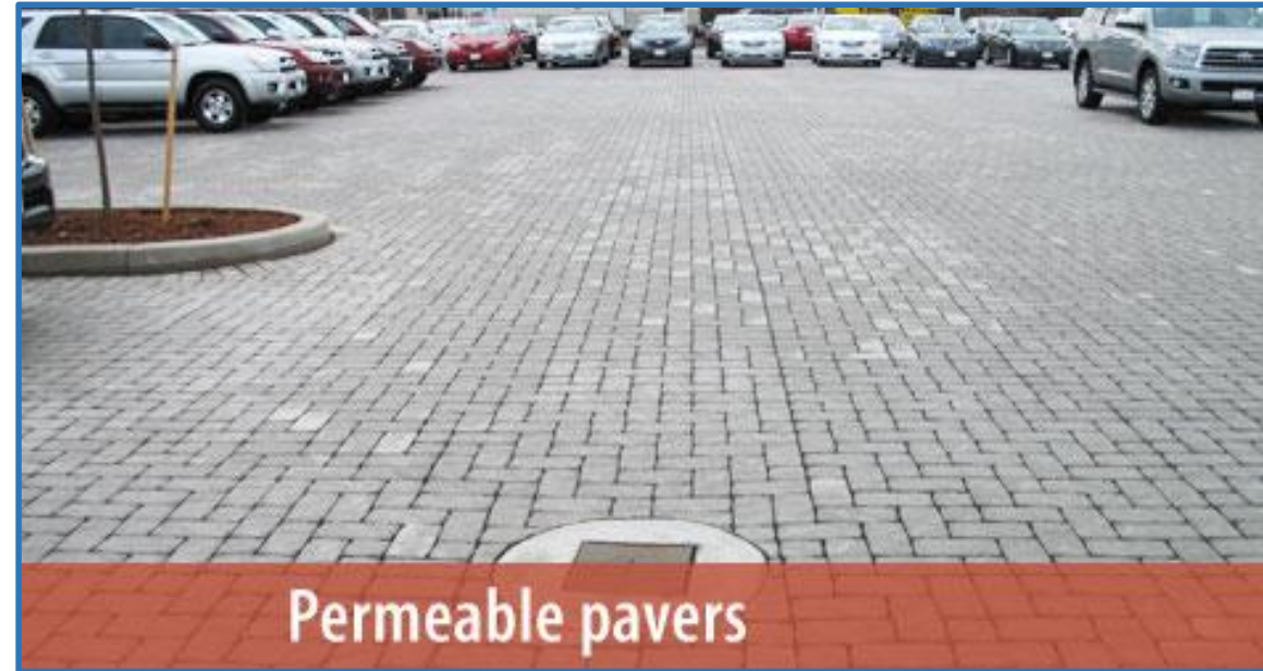
Outdoor Area – Hardscape
