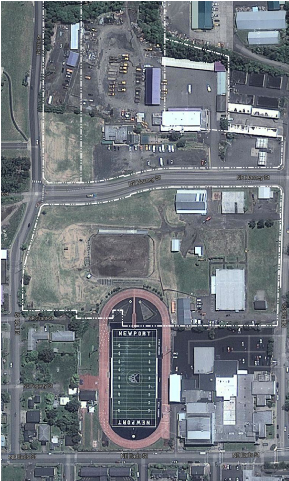
Figure 2. Aerial Image of the Lincoln County Commons
