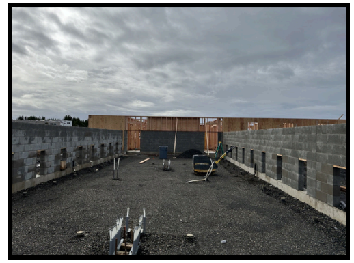
Construction on the new building.
