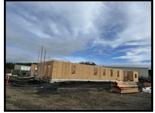
Construction on the new building.
