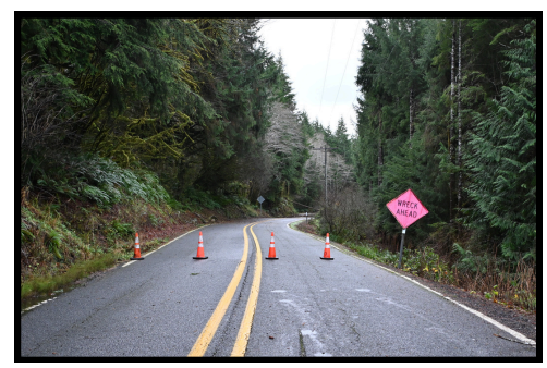
Road closure during Hwy 229 Landslide and winter flooding event.
